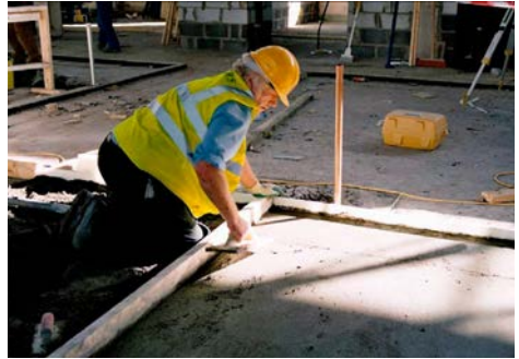
Intensive placement operation of sand/ cement screed installation
