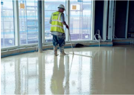
Simplified and less demanding placement of Topflow Screed A
